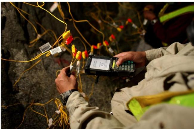
Shotfirer programming the blast. Yellow and red clips indicate the front and rear decks respectively.
